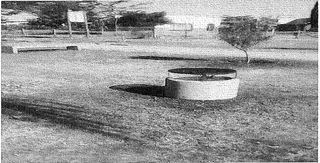
Figure 23 Rehabilitation of an existing park at Lethlabile
